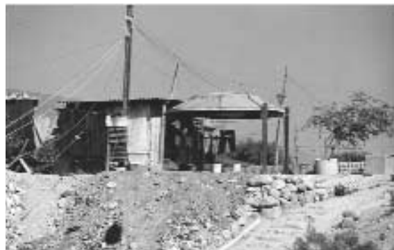
A dwelling constructed out of unused materials, Monterrey, Mexico. A satellite dish is used as a small roof.
