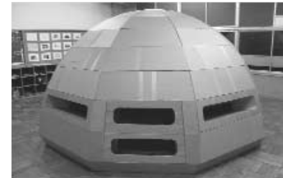
[Paper Dwelling > Learning by Sea Urchin, Model 1:1] is constructed out of cardboard gathered from [Collecting System]. The structure is copying the shell of a Sea Urchin.
